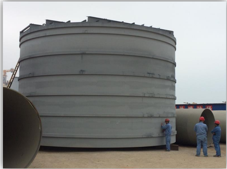
Coal bunkers – 12 huge units of heavy dispensers (63T each) for coal, all fabricated and coated with ZINGA on the Lufeng site.
