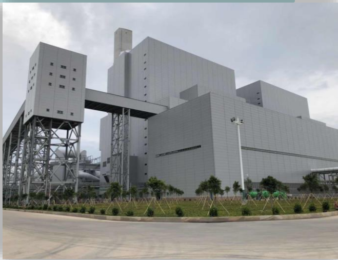
Coal bunkers – 12 huge units of heavy dispensers (63T each) for coal, all fabricated and coated with ZINGA on the Lufeng site.
